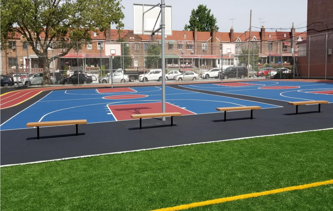
P.S. 151 | TCU Removal & Playground Redevelopment
