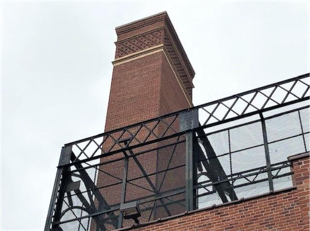
P.S. 69 | Chimney, Gym Floor
